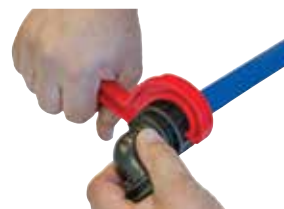
For sizes 40-63, use a nut wrench to nip up the nut a further half turn.
