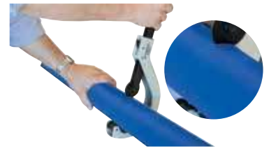
Cut pipe to length with pipe cutters for a clean swarf free finish.
