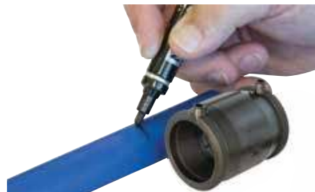
4. Witness mark correct insertion depth.
